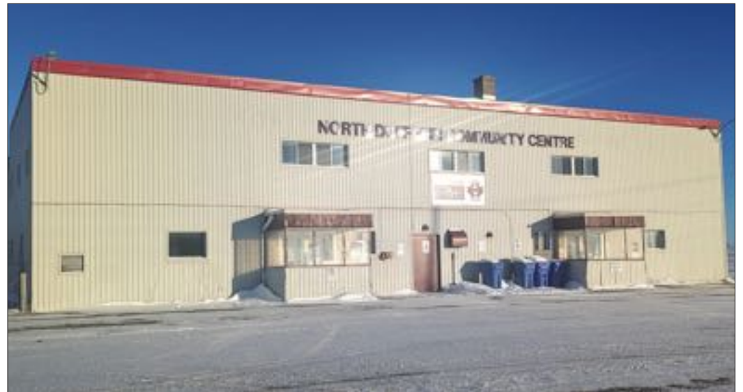
NORTH DUFFERIN COMMUNITY CENTRE
