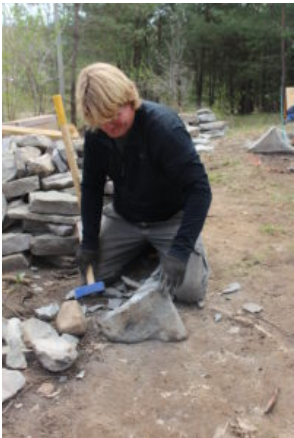
Dry stone work was going on at the mill, and some people came from considerable distance to take part. Torben Larsen came all the way from Vermont.
