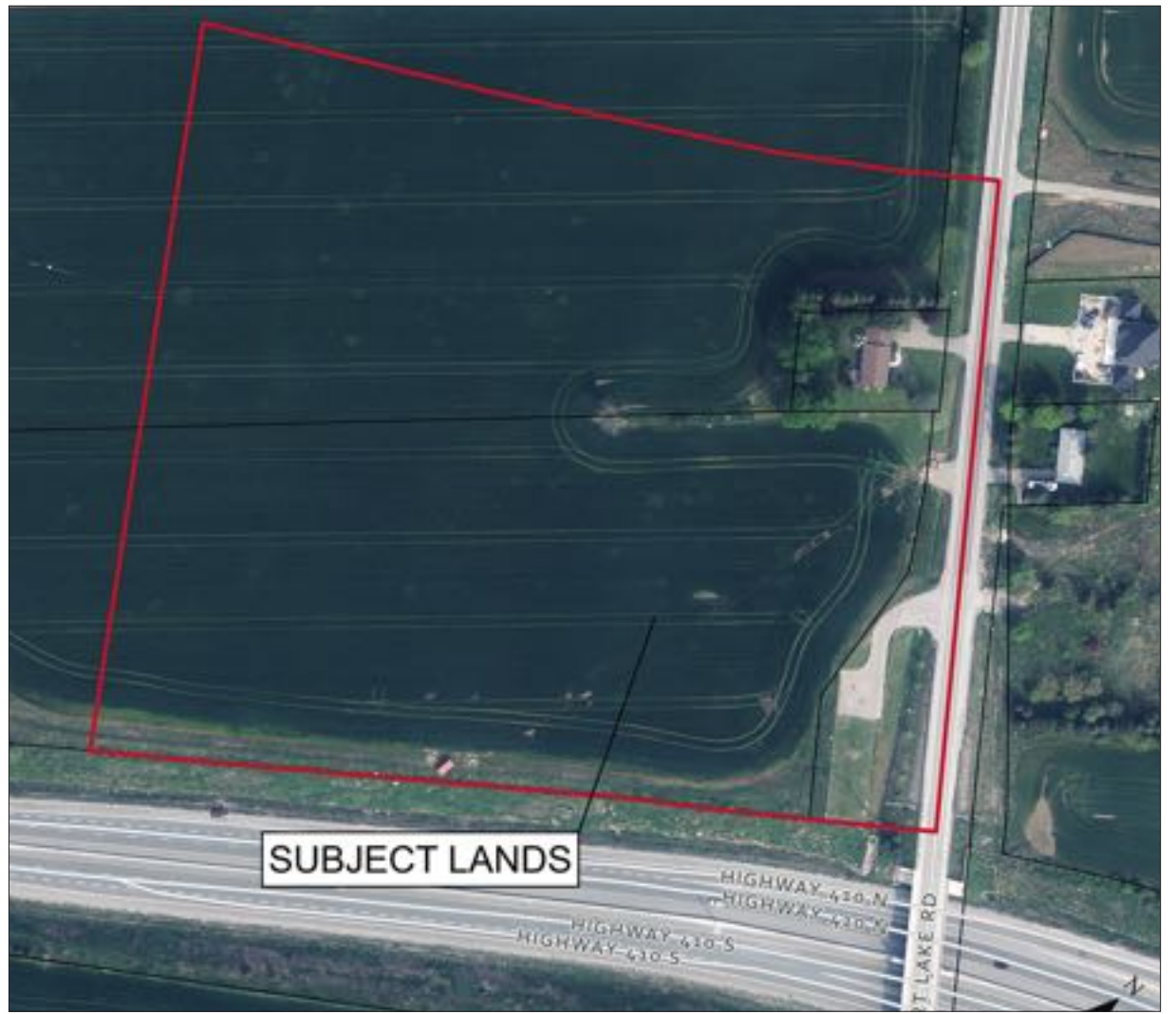
Real estate developer Broccolini plans to create an industrial warehouse and distribution building with ancillary offices here. In order to do so, the developer must extend Abbotside Way to Heart Lake Road.
