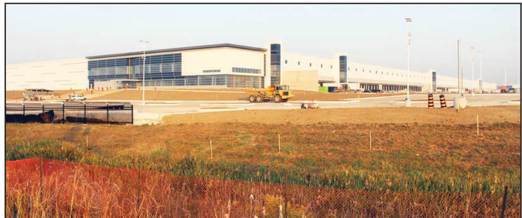
Work is progressing on the Canadian Tire distribution centre at the corner of Coleraine Drive and Healey Road in Bolton.
